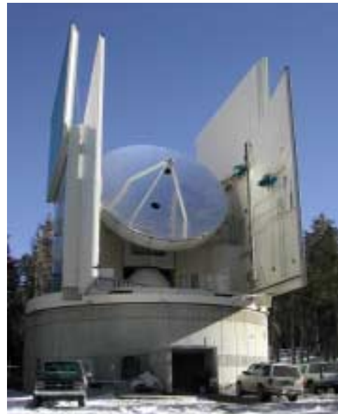
Figure 3. The SMT 10 meter located at Mt. Graham, AZ, the most accurate radio antenna built to date.
