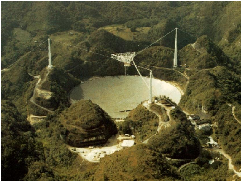
Figure V.A.2: The Arecibo radio telescope. The spherical primary reflector is 1000 ft in diameter. A line feed for 400 MHz operation can be seen hanging below the platform and track. The tip of the line feed is at the paraxial focal point of the spherical primary.
